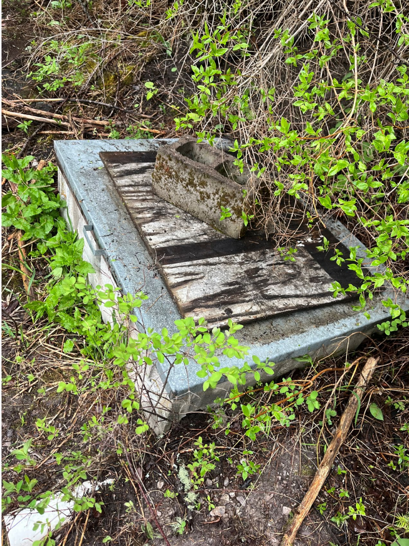
Concrete block spring box with metal shoebox style lid. The black overflow pipe is unscreened.
